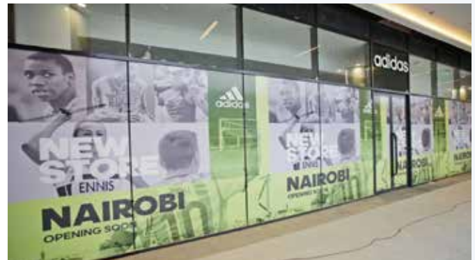
Adidas undergoing the fit out process
