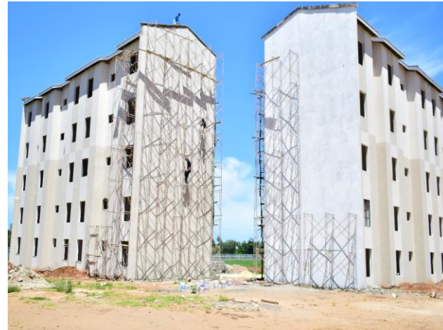
Palm Ridge Expected Completion – Dec 2020
