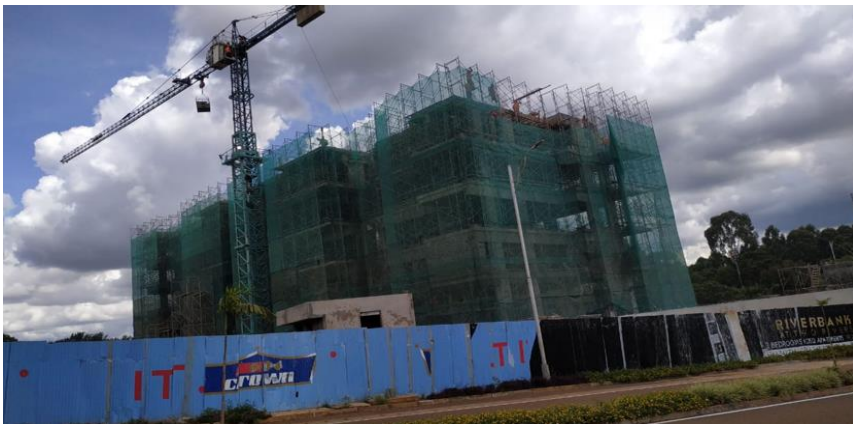
Riverbank Apartments Expected Completion – June 2021
